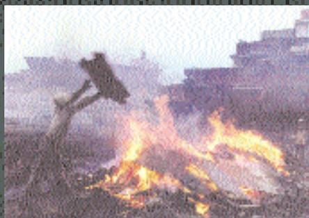
Ship-breaking in Alang, India, where the considerable hand removal of asbestos and open burning of wastes creates severe occupational and environmental hazards.
